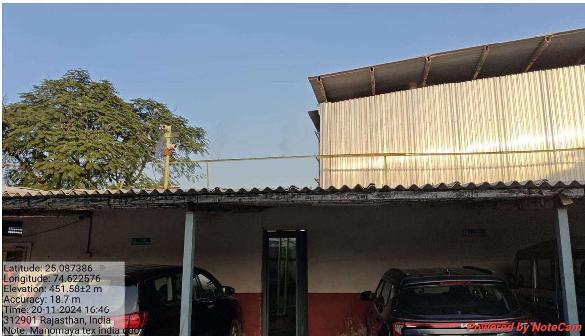
Odor Control System at the entrance
